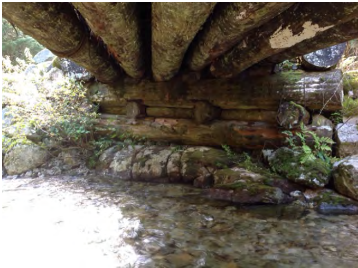
log structure underneath - right bank
