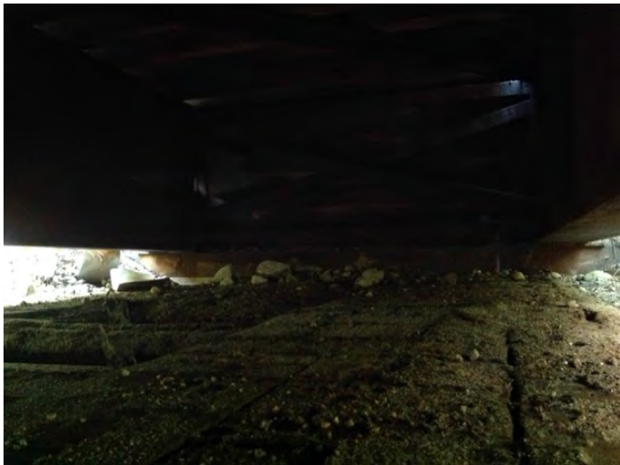
Right Bank Abutment when facing downstream
