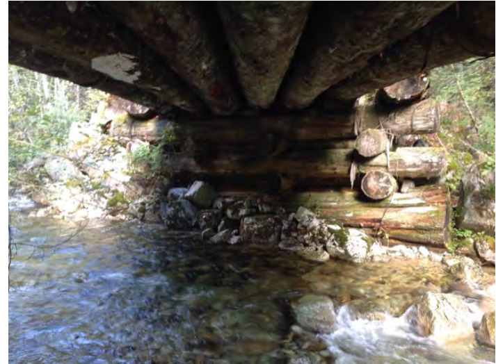
log structure underneath current - left bank
