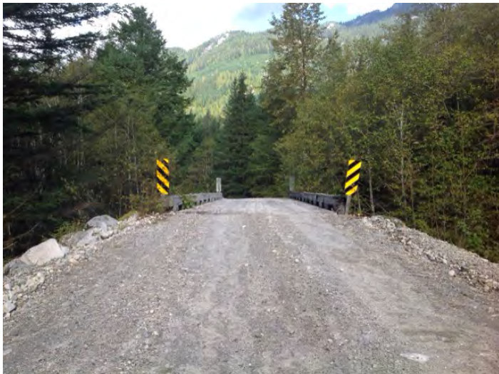
Approach from Right Bank when facing downstream
